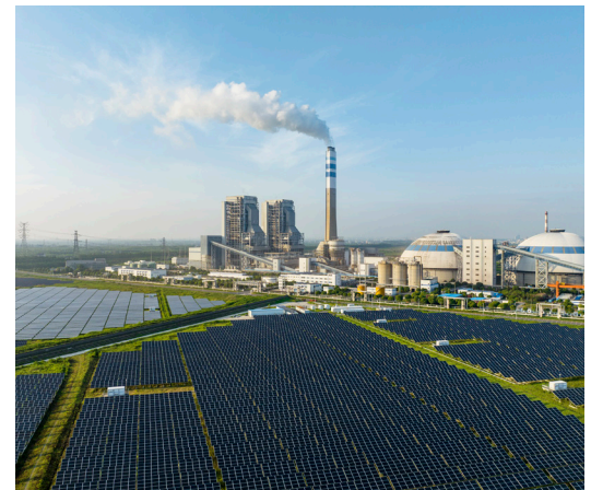
Thermal power generation and solar power station in Shanghai, China./Gettyimages
